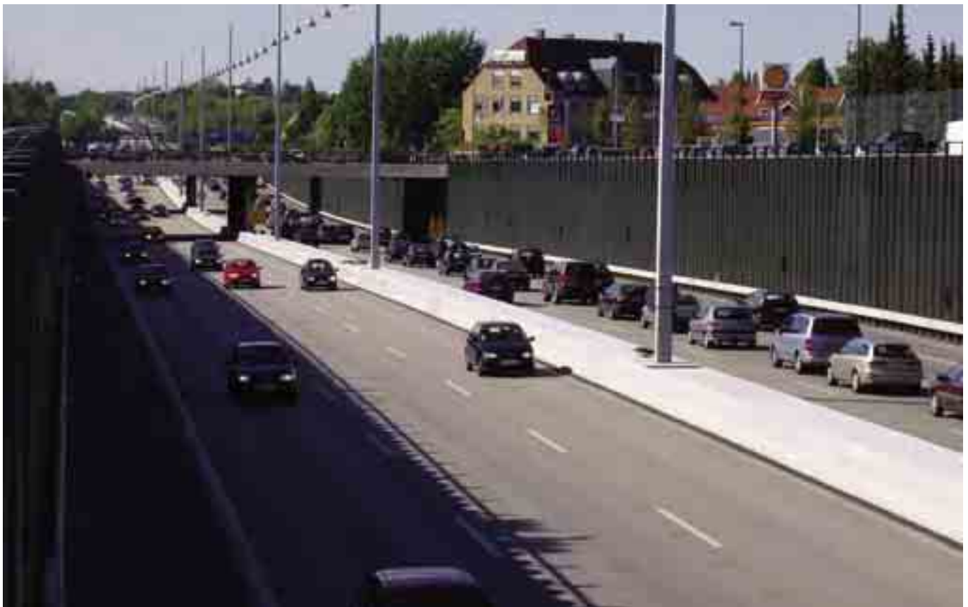
The white concrete crash barriers brightly separate the oncoming traffic. A functionality, which is maintained in dark and rainy weather. The above illustrates an example from a highway in Denmark.
