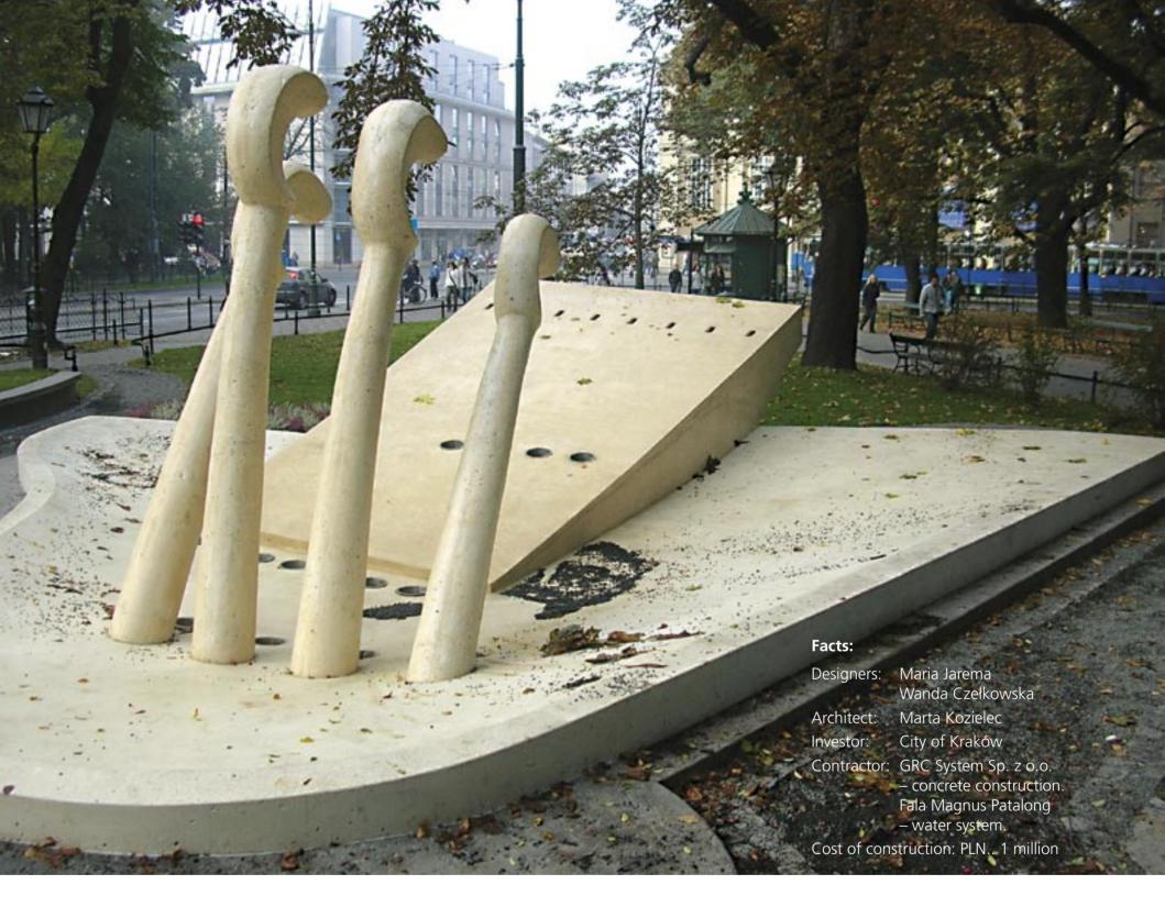
In this case white mortar was coloured with a yellow pigment. The use of AALBORG WHITE® cement and alkali-resistant glass fibres in concrete produces satisfactory technical and aesthetic results. It is also a very interesting solution for the water circulation system in the fountain – water sprinkles from a "piano lid" creating 8 strings and also from hammers which are opposite to it.
